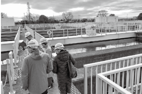
▶行田浄水場の薬品沈下池
